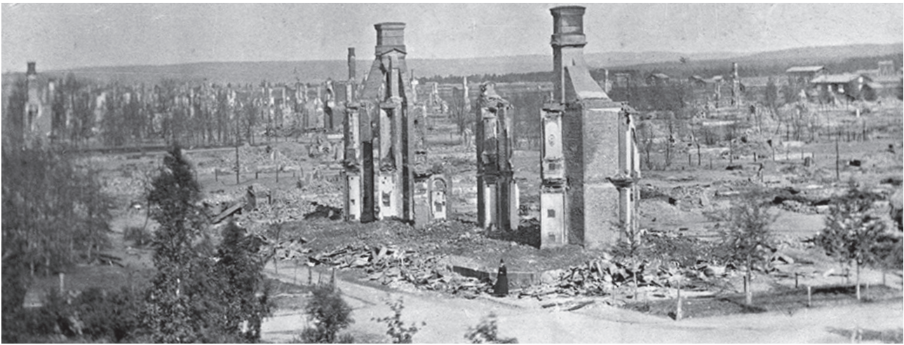
Figure 3. Photograph from the prison towards the devastated town. Remaining chimneys from houses nearby stand. Source: Umeå400 webpage
